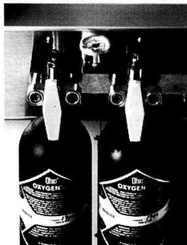
Figure 6-6 Oxygen Yoke and Regulator Assembly (see list on 6-1 and 6-2)
